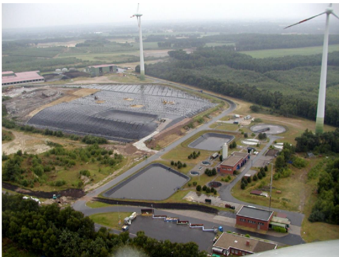
Figure 1 Disposal centre Wilsum from a bird's eye view
