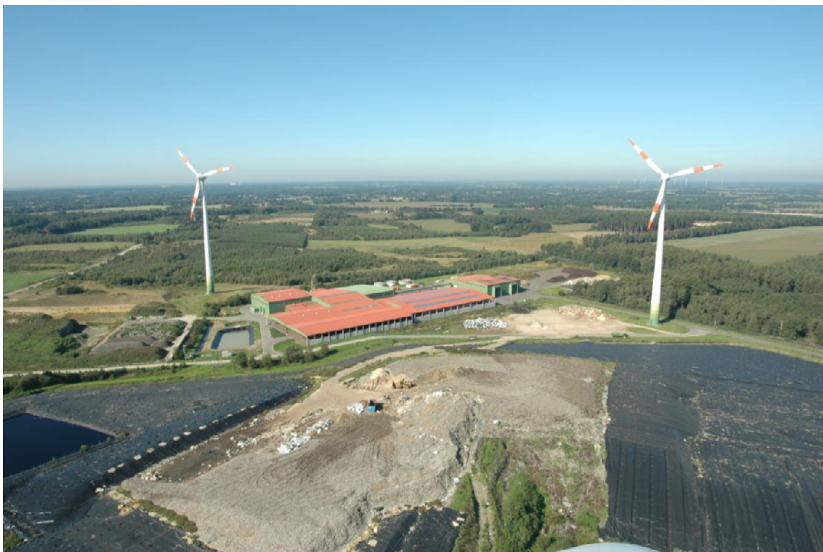
Figure 1 MBT plant Wilsum
